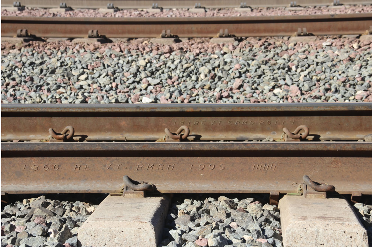
A close up of the rail at Summit. Note that the inner rail which receives much of the lateral weight of the train cars' wheels, as the train go through this bend, is 141-pound rail while the outer rail, which receives less of the train's lateral weight, is 136 pound rail
