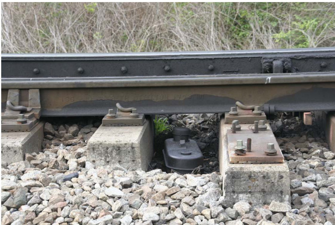
A kerosene heater rests under the switch points ready to heat the rails this winter.
