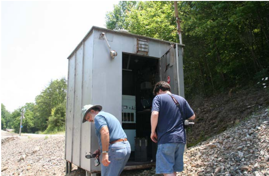
The daylighted Lebanon Branch Tunnel #5 with its equipment dragging detector box. The abandoned Tunnel #5 is buried in the hillside to the right.
