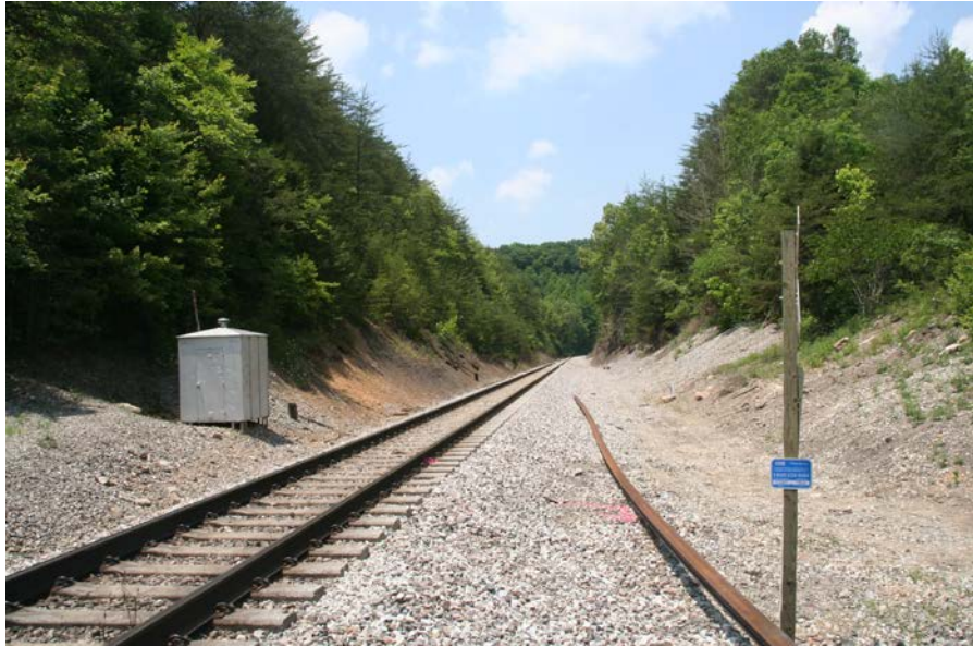
The daylighted Lebanon Branch Tunnel #5 with its equipment dragging detector box. The abandoned Tunnel #5 is buried in the hillside to the right.
