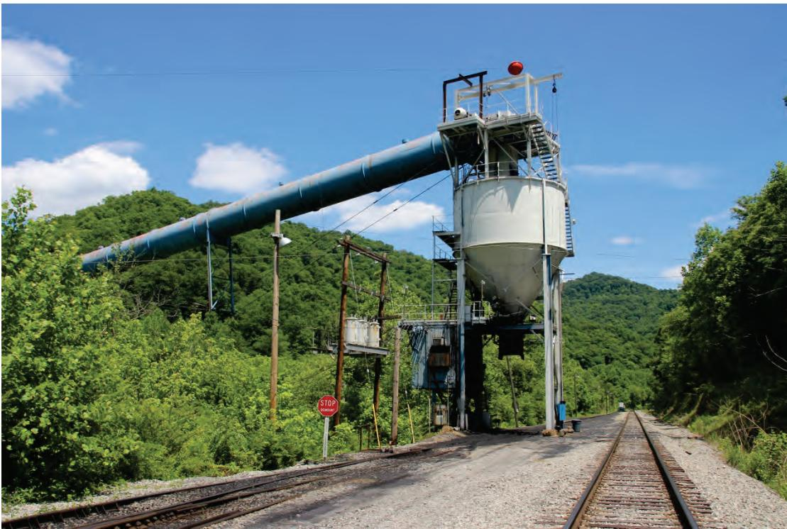
Above and below: Located at CMP 9.5 on the Coal Run Subdivision is the Scotts Branch Mine coal tipple owned by Excel Mining. The tipple loads a train once a week. The tipple has its own mine goat, JDNX 2001, a cableless ALCO locomotive. Note the operator's platform to the left of the front coupler.
