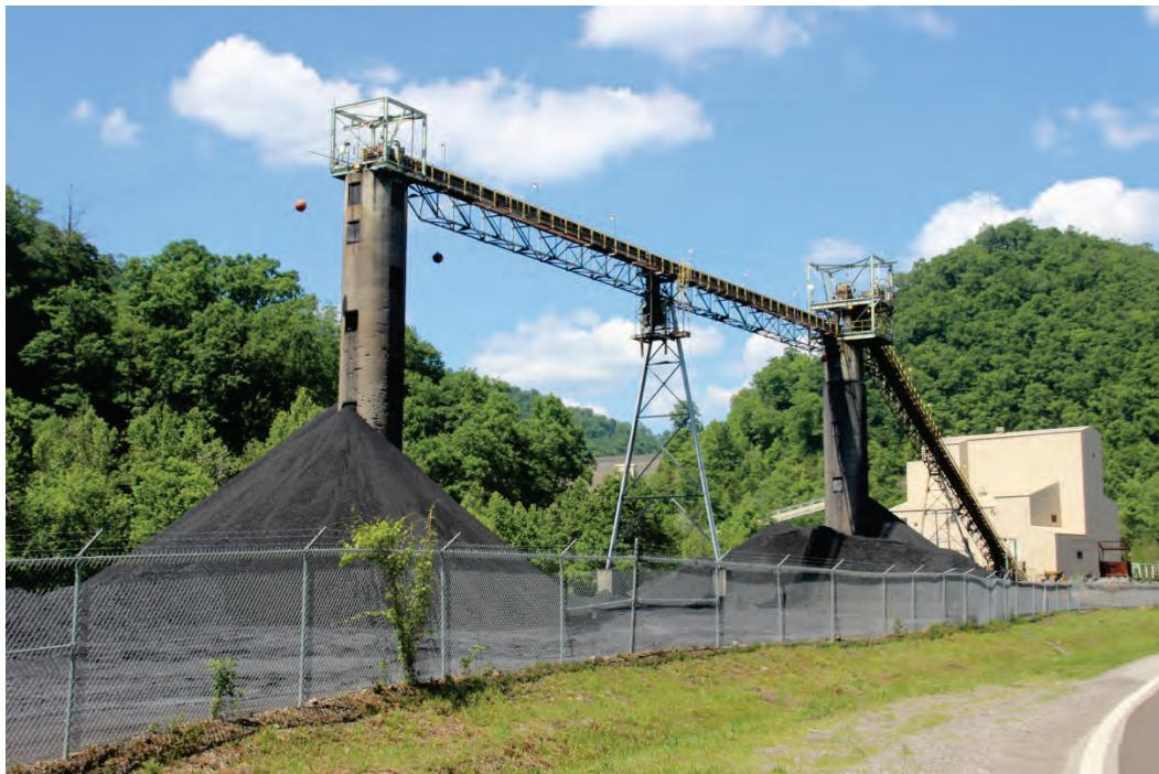
Located near the end of the Coal Run Subdivision is the High Ridge Mining Coal Preparation Plant and Coal Loadout. Coal is seen here being carried by conveyor belt from the preparation plant to the coal stockpile. From here it will be transported by another conveyor belt to the tipple. The CSX siding name is "Goff."
