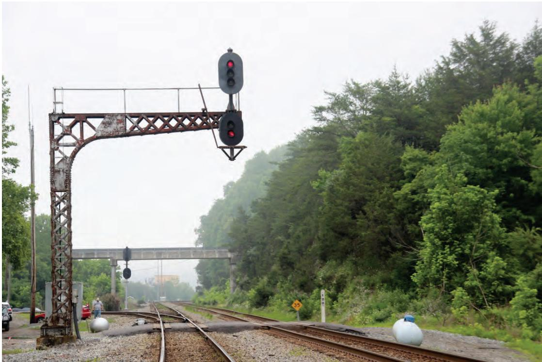
**Looking south from the CSXT main at Coal Run Junction. The cantilever signal protects the track on the left that leads into Coal Run Yard and Coal Run Subdivision.**
