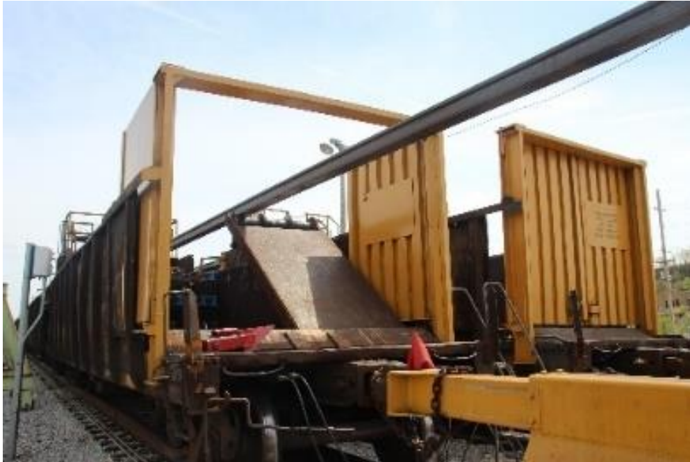
The ribbon rail being guided into the rail carrying car
