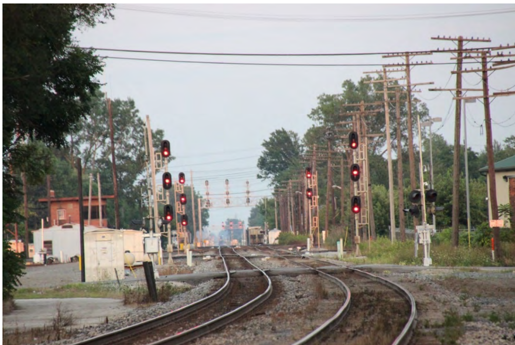
This view looking toward F Tower from the former B&O Passenger Depot shows the various signals an eastbound CSXT train encounters as it approaches the diamond at the now closed F Tower.
