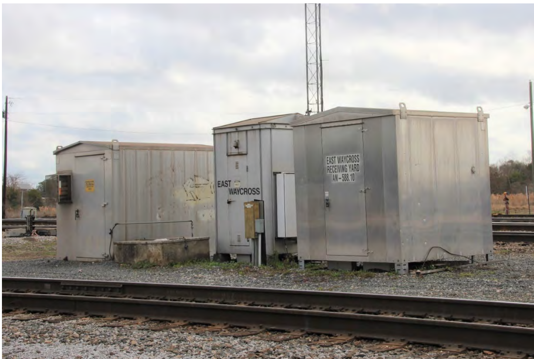
These mechanical boxes are the replacement for the tower that once controlled the diamond and wye at the east end of Rice Yard.
