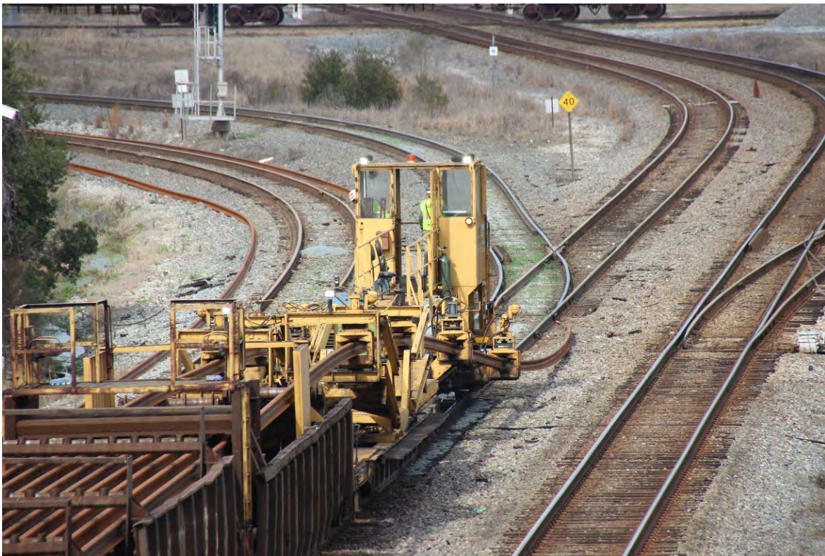
The CSXT crew of RAUN 10 is starting to lay continuous rail. Note the rail coming off both sides of the gondolas and being placed on the ground next to the rails to be replaced.
