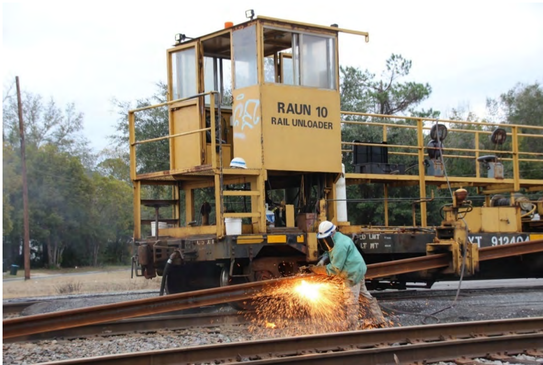
The torch man is cutting the ribbon rail just short of the highway crossing.
