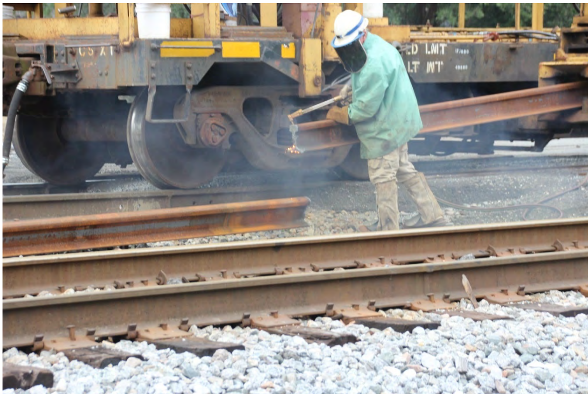
The torch man is cleaning up the cut in preparation for the relaying of the ribbon rail on the other side of the highway grade crossing.
