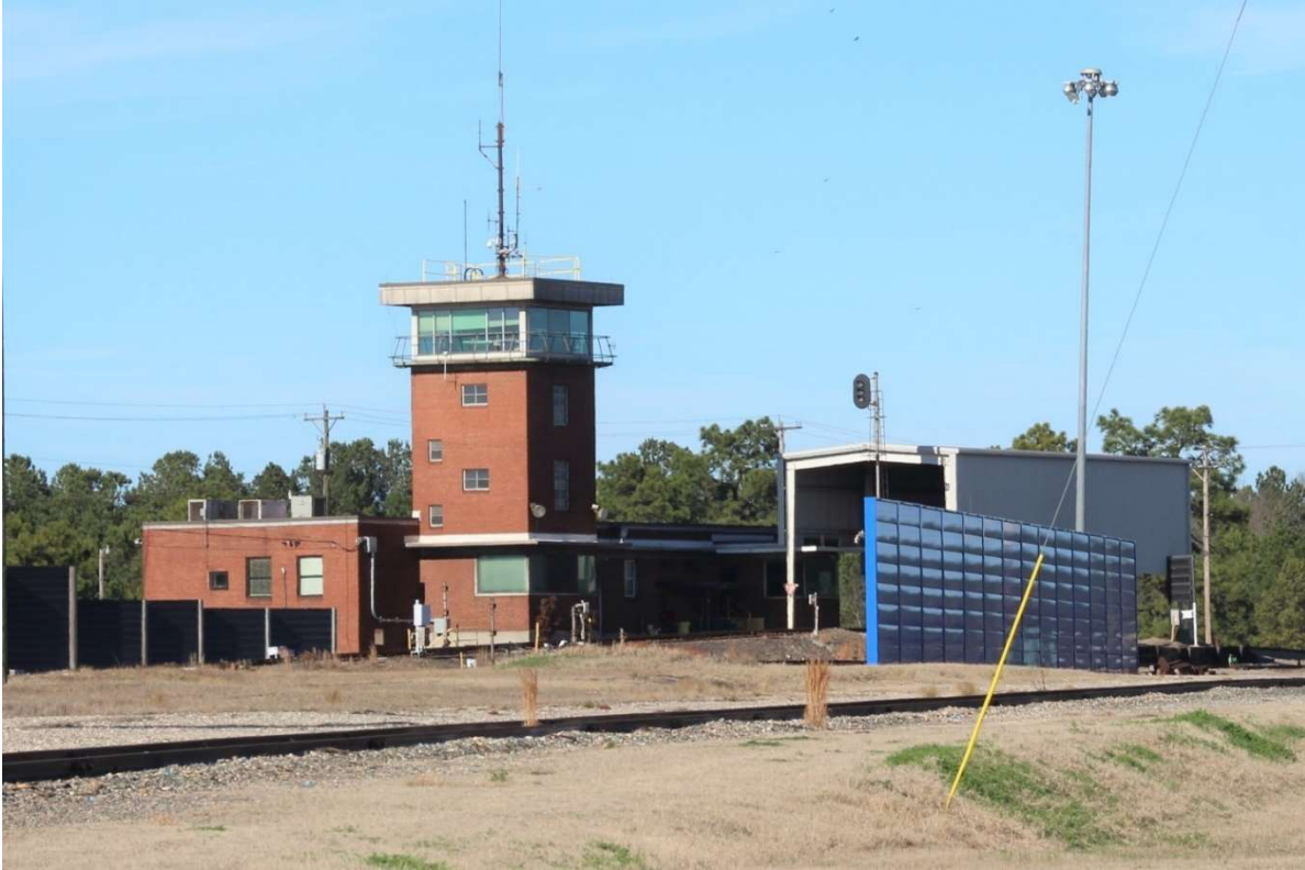
A view to the northwest of Tower A showing the sound barrier to protect those east of the hump from the squeal of the cars going through the retarders.
