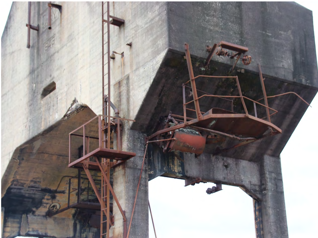
Above and below are views of the remains of the coaling chutes support metal work.
