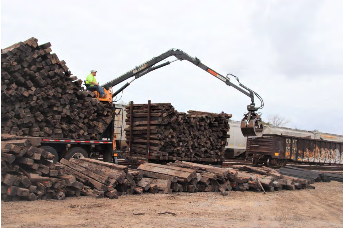
A cherry picker crane is being used to pick up the old ties for loading onto a trailer for removal to a disposal site.
