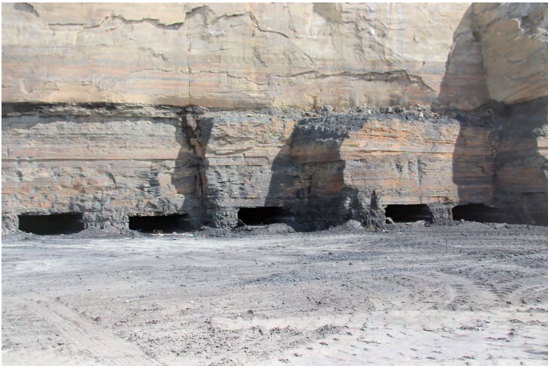
A close-up view of the shafts from the highwall that tunnel back into the coal seam.
