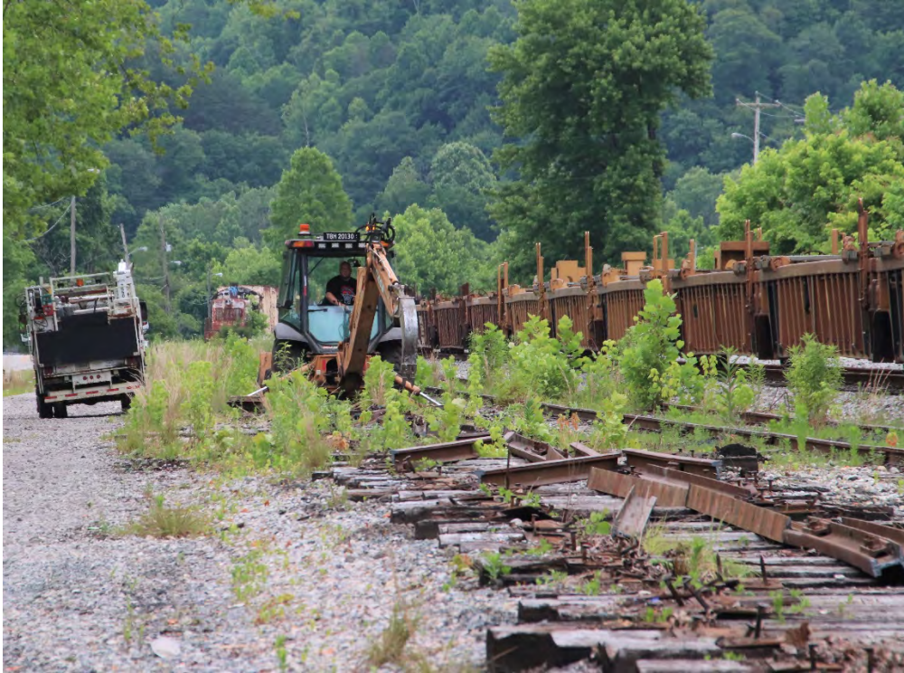
The CSXT crew at work removing the yard track
