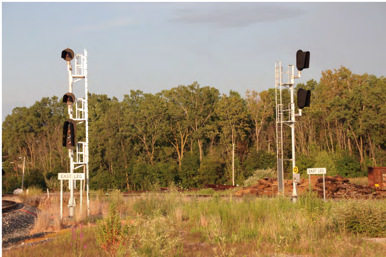
Both signs by the two signal towers read “East Leg.” Note the derail warning sign on the right signal tower.
