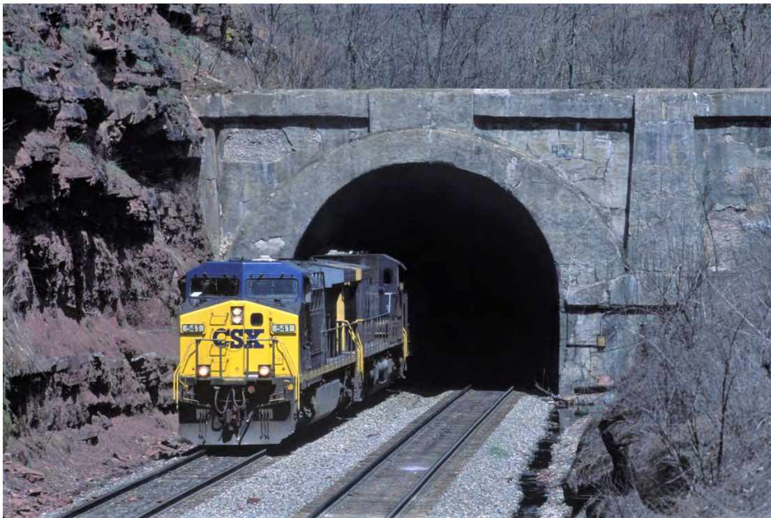
CSXT 541 is seen westbound exiting the 4,000-foot-long Sand Patch Tunnel located at Sand Patch, Pennsylvania. This double track tunnel was opened in 1912 by the Baltimore & Ohio Railroad to replace the line's original 4,777-foot single track tunnel.
