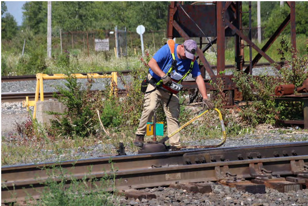
The Trainman now throws a different switch so as to direct the next car into the correct siding.
