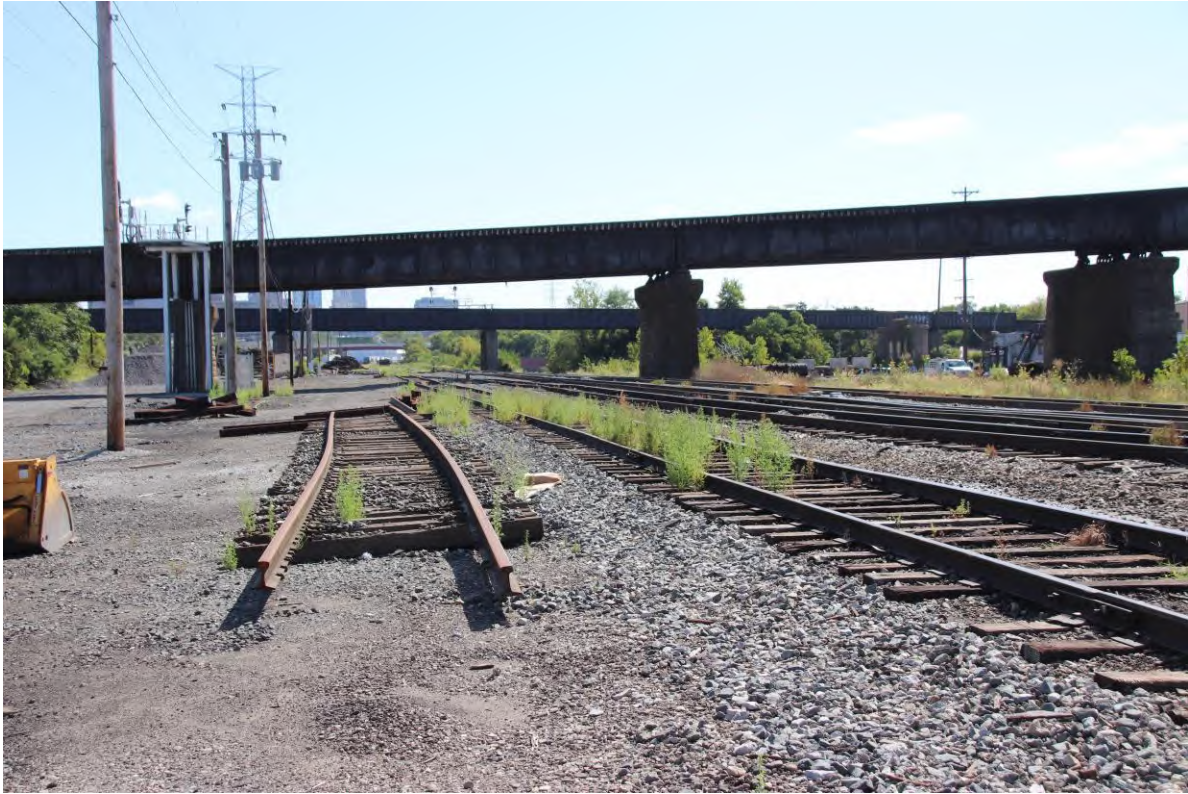
Track in the process of being taken out.
