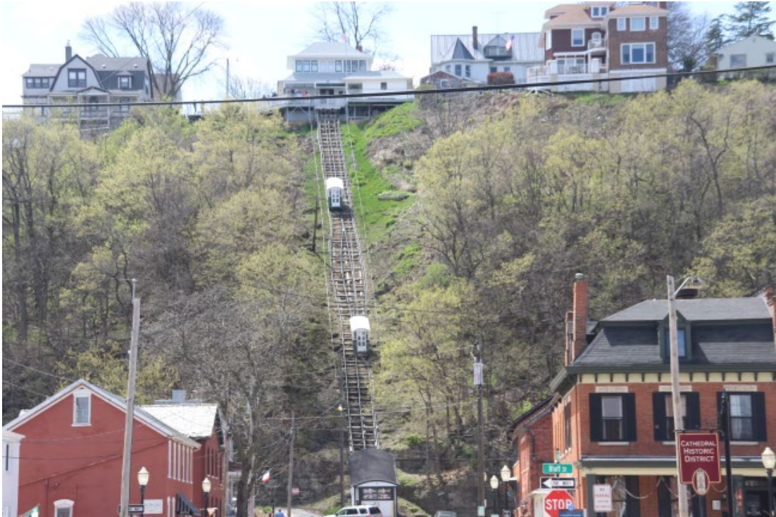
View from Fourth Street looking up at the head house. The house to the left of the incline is the residence of the owners of the incline.
