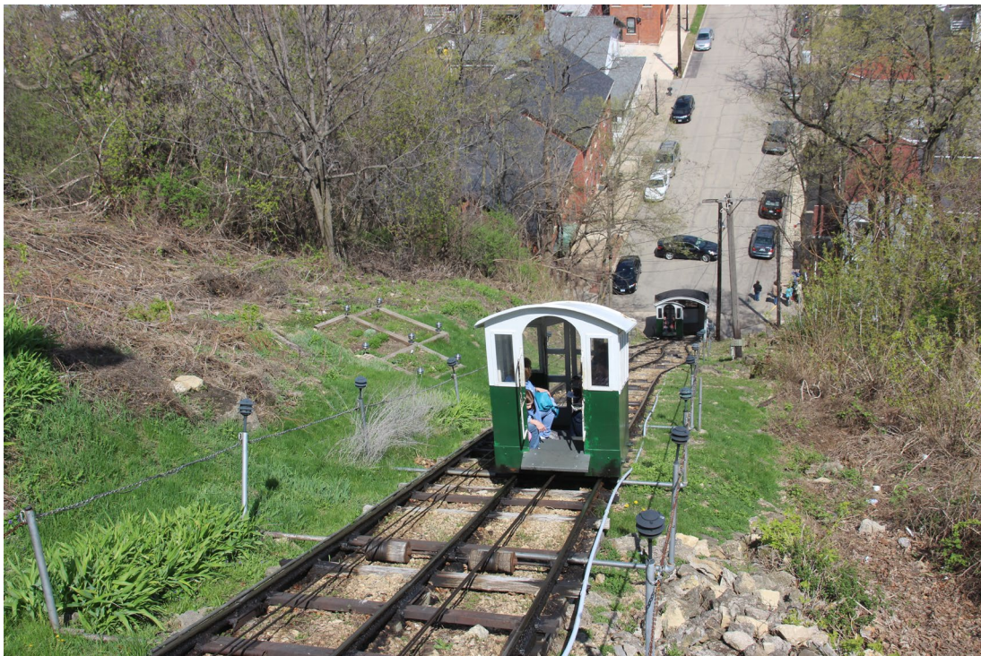
A view from the head house down toward the lower level boarding platform. Note that while the downhill side of the car has a door closing the car, the uphill side has only an opening.
