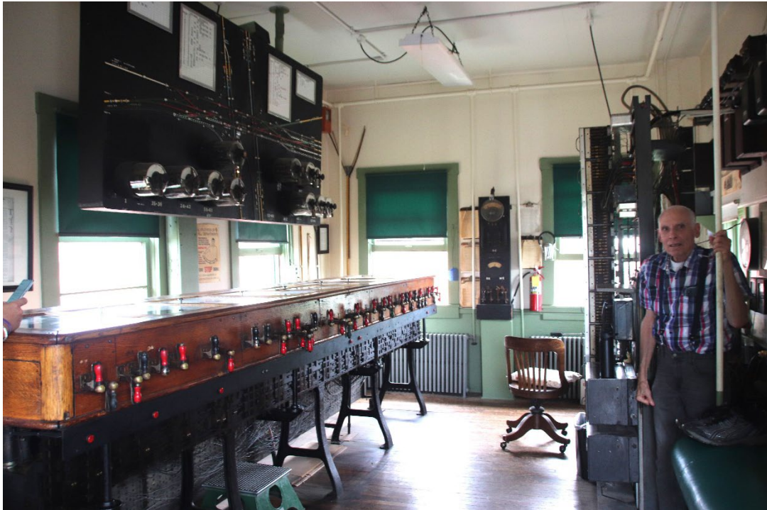
Inside AC Tower
