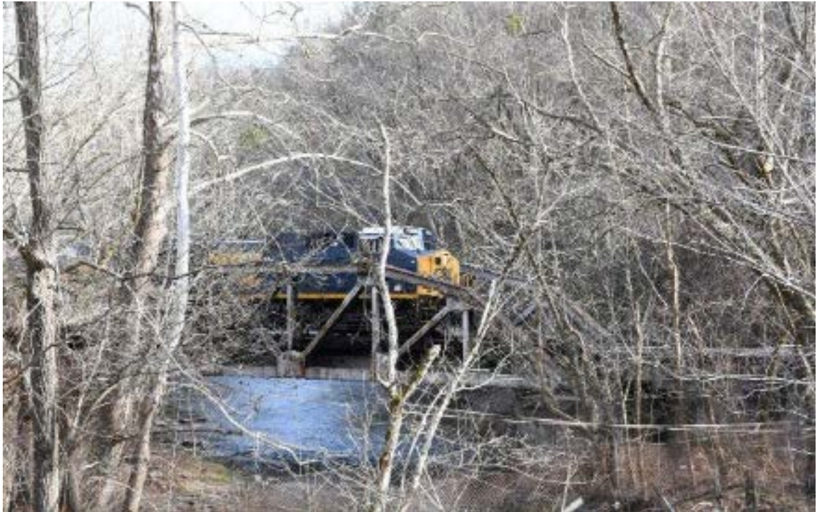
R615-29 crosses a deck truss over Martins Fork of the Cumberland River at Farmer's Mill.
